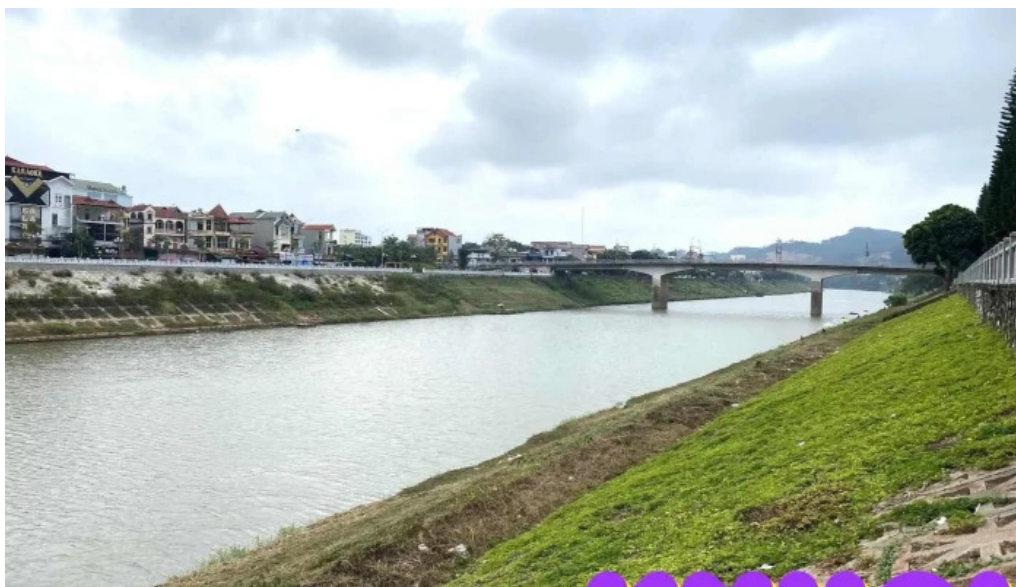
Cau ky cung cau
